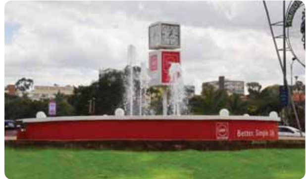
Rehabilitation and beautification of Nairobi Road Island: Kenyatta Avenue, Uhuru Highway Roundabout.
